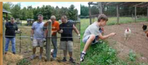
Volunteers from Kennametal help to install fencing around the pasture.
